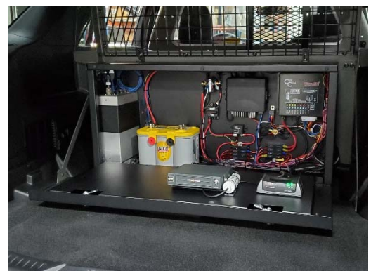
Installation is now complete.
